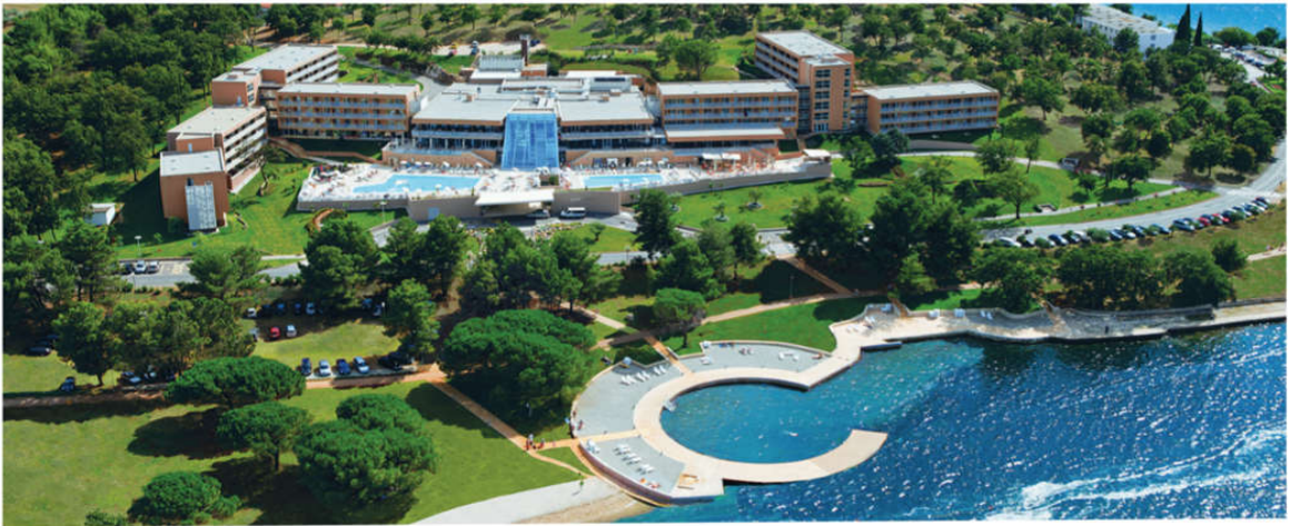
Hotel Molindrio after reconstruction
